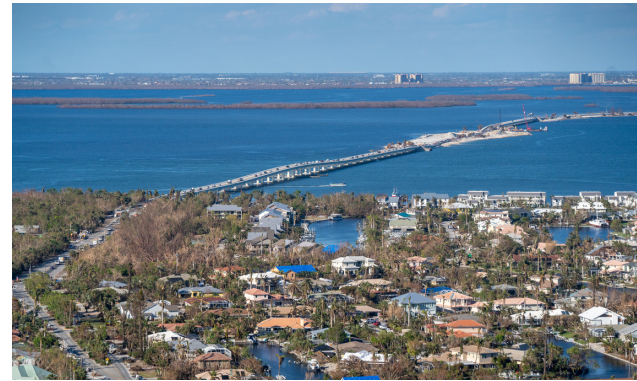
Aerial view of damage to the Sanibel Causeway and surrounding residential homes
